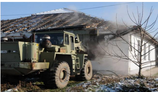
Picture 5 Demolition of Public Health National Institute in Kraljevo damaged in earthquake in December 2010
