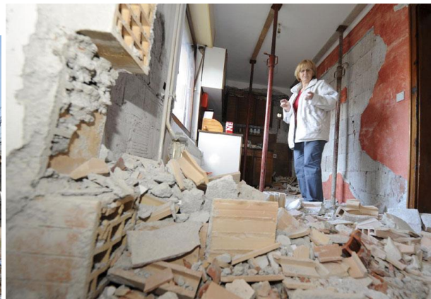
Picture 6 Facility damaged by earthquake, Kraljevo, November 2010
