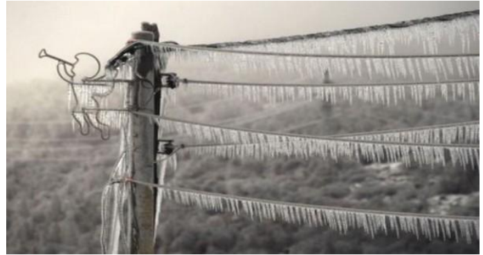
Picture 2 Power line in the area of Majdanpek, December 2014
